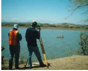
Figure 7 Bathymetry Survey in 2011 and Great storage Changes in Poechos Dam
