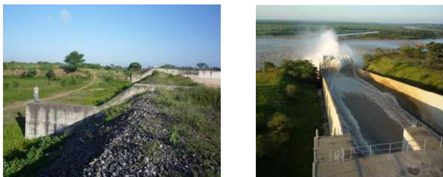
Figure 6 Emergency spillway (fuse dams) and spillway with gates in Poechos dam
