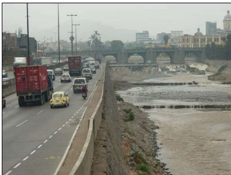
Figure 3. Construction of the Pan-American Highway By Pass narrowed the Rimac River. Notice the railroad fill on the left bank of the river. The photograph was taken looking in the upstream direction.
