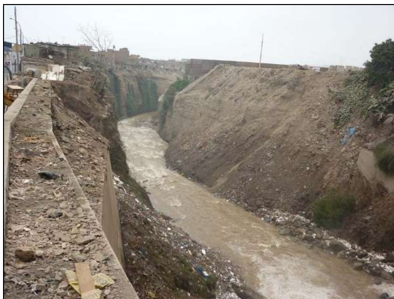
Figure 2. Urban canyon downstream of the Army Bridge.
